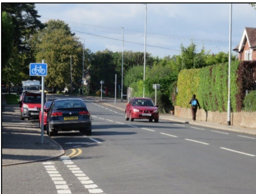
Cars are frequently parked within the cycle lane
