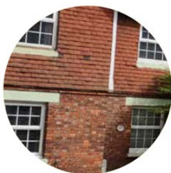
Hanging tile and patterned brick
